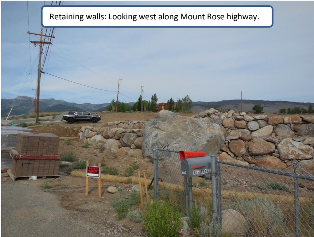
The boulder in the center of the preceding photo is a part of the lower of the two retaining walls and it approximately 7 feet in height above ground level. The plans submitted by the applicant with this request for a Special Use Permit include reducing the above-ground height of that portion of the retaining wall to 4 feet. Within the front yard setback area, fences, walls and perimeter plantings of 4 feet in height are permissible. The plan detail on that area follows:
